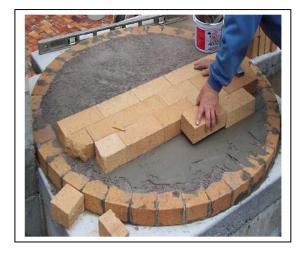
3) Set the entrance tunnel (2 pcs) and wall sections (2 pcs) as shown using HeatStop II refractory mortar.
