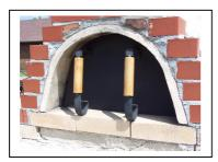
5) Parge dome with insulating refractory concrete at least 2" thick. Fill cores of side sections and entrance sections with insulating refractory concrete
