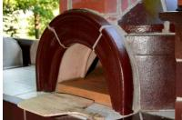
8) A door-without-a-hinge or entrance cover for the oven entrance is provided. It can be propped up slightly (to provide combustion air) at the outside of the entrance when a fire is burning in the oven and can be pushed in farther against the seat in the tunnel to close off the flue to keep the oven warm longer after the fire has burned out.
