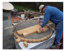
3) Lay out a 36" circle on oven floor and set the entrance tunnel and base sections using HeatStop II refractory mortar.
