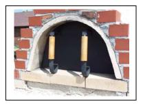
5) Parge dome with insulating refractory concrete at least 2" thick. Fill cores of side sections and entrance sections with insulating concrete
