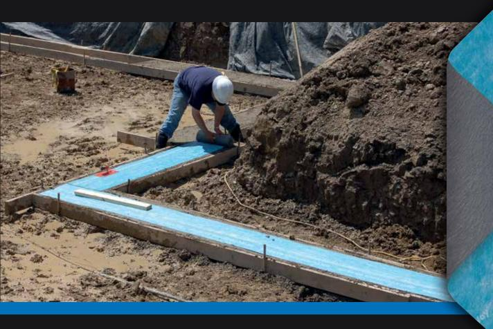
Resists capillary rise of moisture in foundations.
